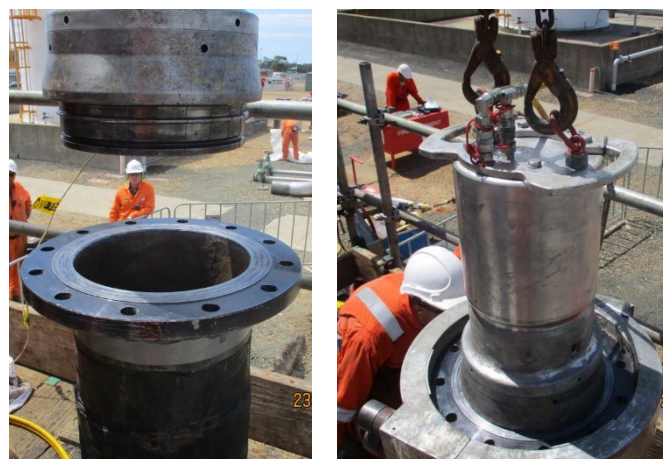
Quickflange tool alignment and setup
