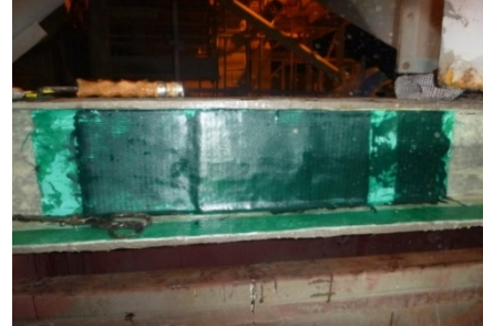
Application of Technowrap™ SRS to web of I-beam
