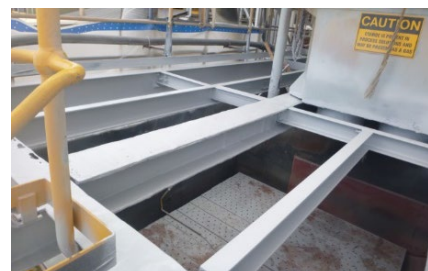
Complete Technowrap™ repair with client specified protective coating
