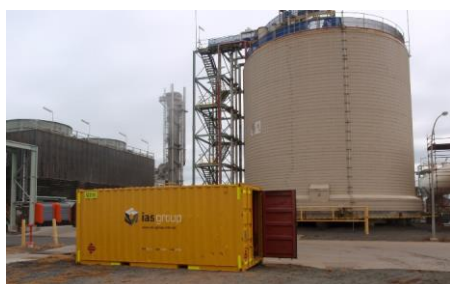
Ammonia Tank Roof Repair
