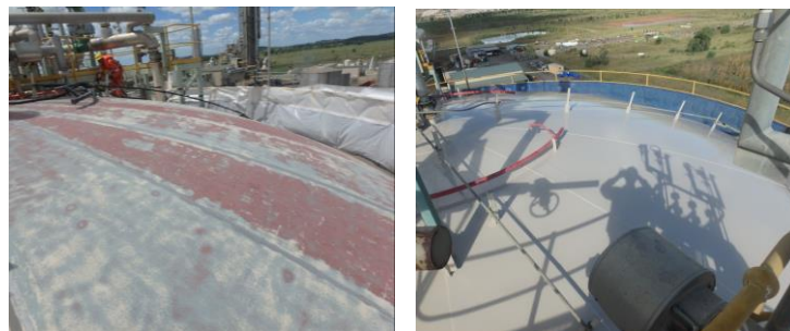
Before and After Tank Roof Refresh
