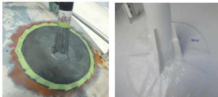
Technowrap™ Roof Patch Repair
