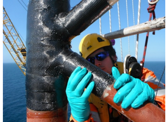
Application of Technowrap™ SRS
