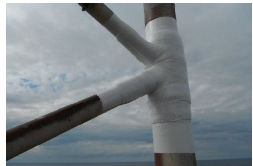
Completed Technowrap™ SRS repair with coating
