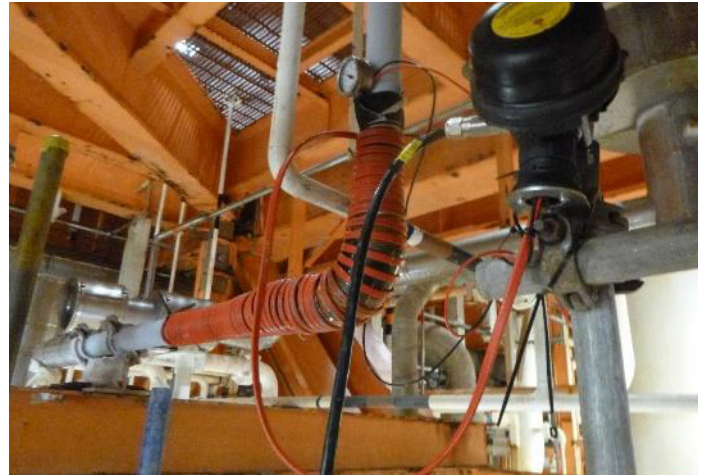
Temperature-controlled heat tape was used for careful control of the resin curing process
