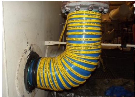
Post curing of repair via heat tapes
