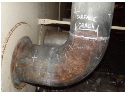
Repair location before surface preparation
