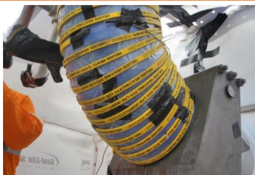
Heat tape to assist with cure speed
