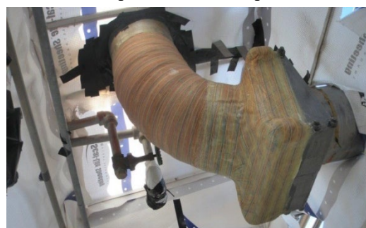
Technowrap 2K™ HT completed repair
