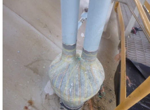
Profiling and initial layer application
