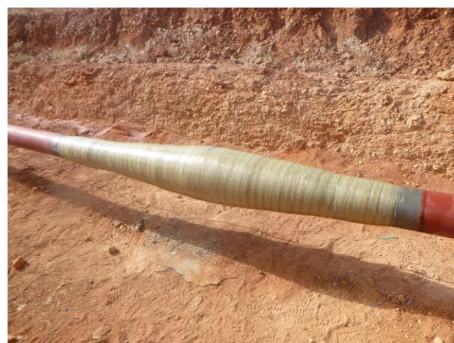
Completed Technowrap™ Repair
