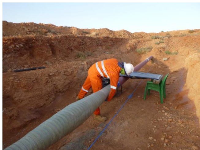
Application of the Technowrap™ Repair
