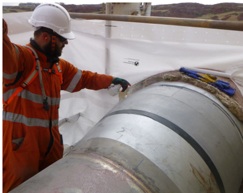
Surface preparation complete
